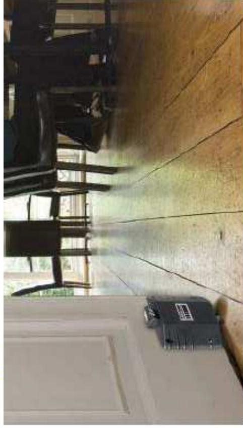
We've all seen or done it before! A fire door wedged open on a hot sunny day or the fire door propped open so that people can easily pass, however it is illegal and dangerous to do this, in fact it is a direct contravention of Fire Safety regulations in the UK. In the event of a fire, this hazardous practice will result in the fire spreading quicker, causing more damage and putting people's lives at risk.
